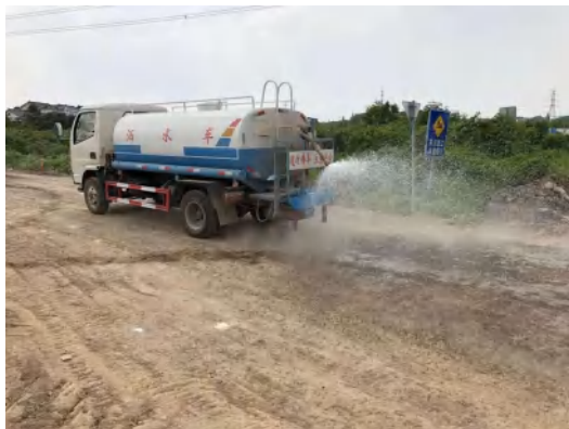
施工期洒水抑尘
